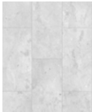
R109 PT Concrete
